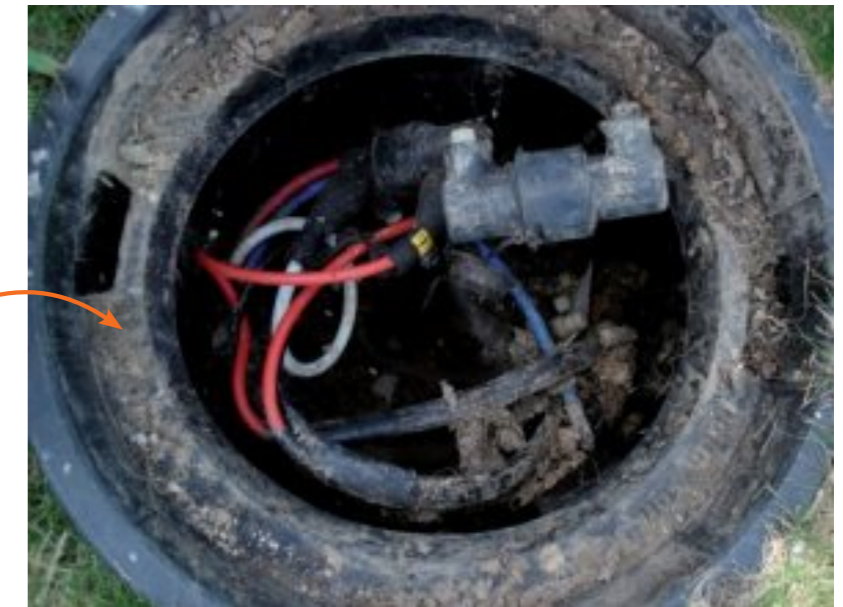
K199 - Installation in a pit
