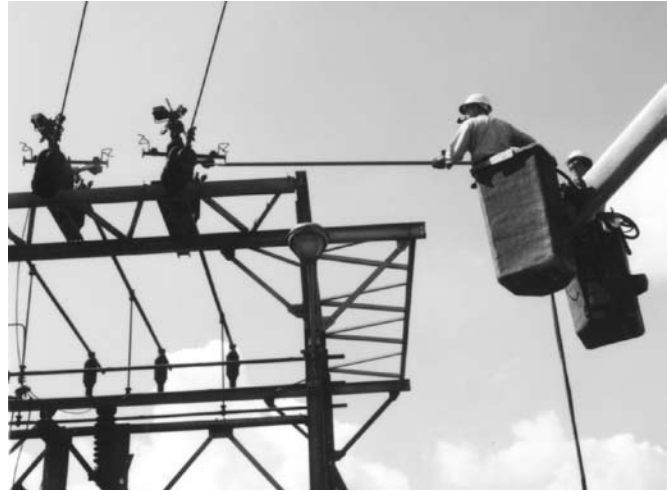
Cleaning substation insulators and suspension insulators.
