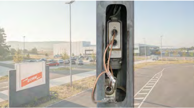
Earthing and short-circuiting device installed at a junction and fuse box of a street lighting mast
