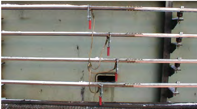
Three-pole earthing and short-circuiting device with screw clamps.
