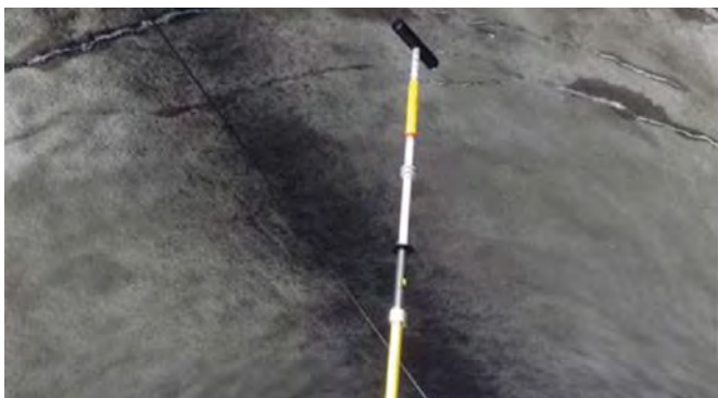
Removing icicles on a tunnel entrance.
