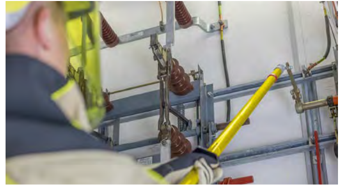
Switching a disconnector by means of an SCS switching stick
