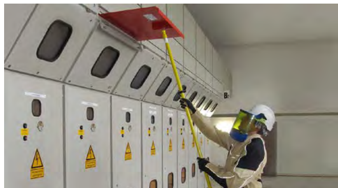
Inserting an insulating protective shutter (type A3) by means of an operating stick
