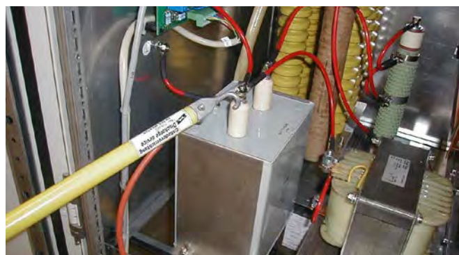
Single-pole device for discharging static charges
