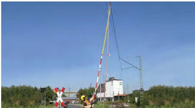
Attaching a railway earthing device.
