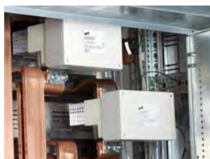
Quenching device above the supply switch
