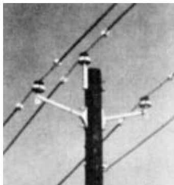
Three Phase Pole Top with APD Lightning Protectors in Place. (Only one unit is required on the load side of the line at each support for a radial circuit)
