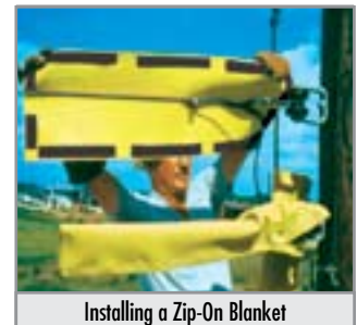
Installing a Zip-On Blanket
